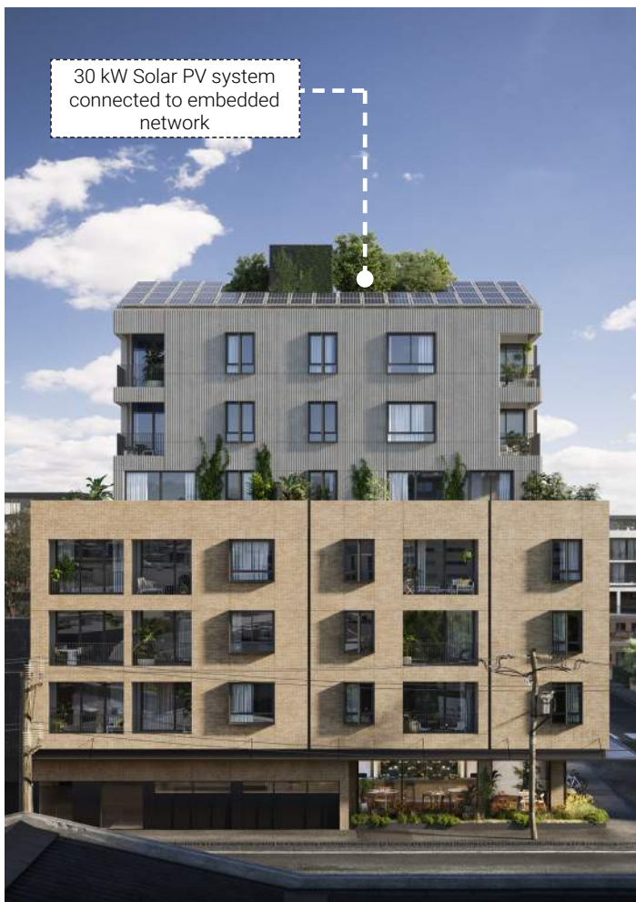
Figure 2: Solar PV System - Breese Street
